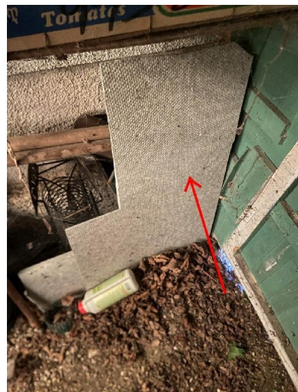
Local 02. Plaque fibre-ciment.
