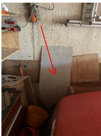
Garage 01. Plaque fibre-ciment.
